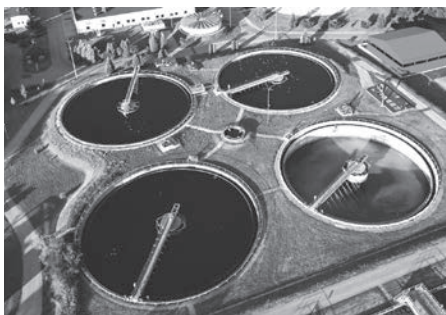
Water treatment system
